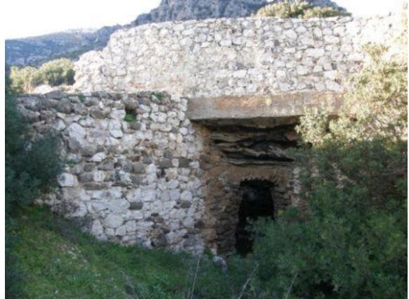
F1 Old furnace in the territory of Siniscola
